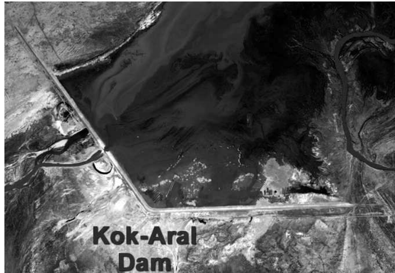
Figure 6. New Kok-Aral dam built by Russian company “Zarubezhvodstroy” in 2005
